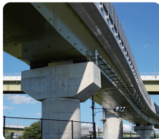
Highway Side Walls
