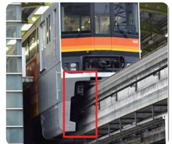
Guide Rails of Monorail Tracks
